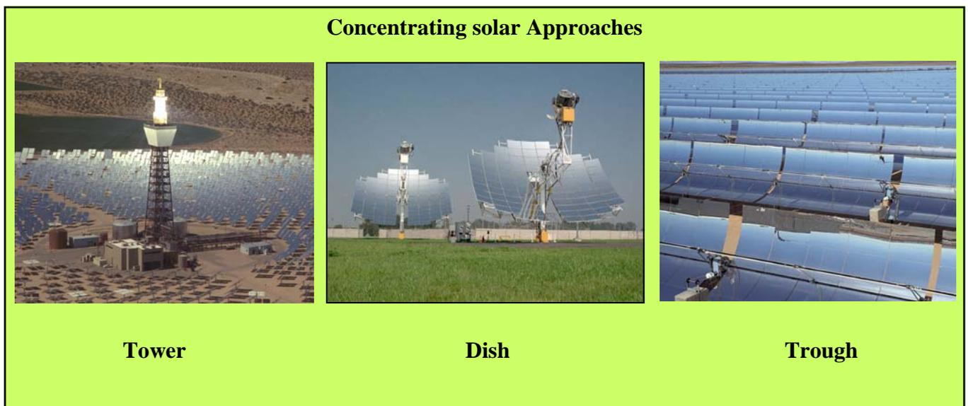
Figure 1 : Solar tower, dish and trough power plants
