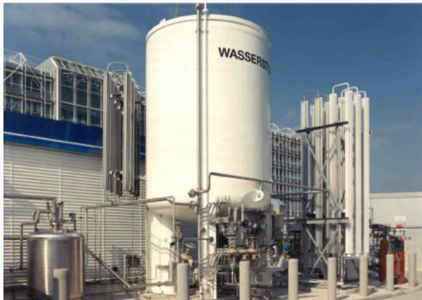
**Figure 3: Linde liquid hydrogen tank plant**
