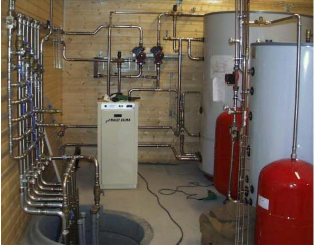
**Figure 6: A view of the storage tank and the piping inside the thermal cottage**
