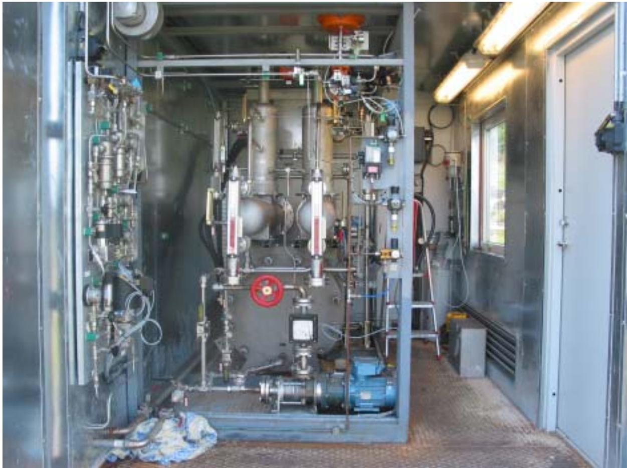
Figure 8: The 50 kW high-pressure alkaline electrolyser
