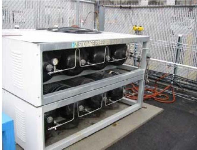
**Figure 3: 438 bar hydrogen station storage bank consisting of carbon fibre composite cylinders. The storage bank allows the vehicles to be fast filled with hydrogen**
