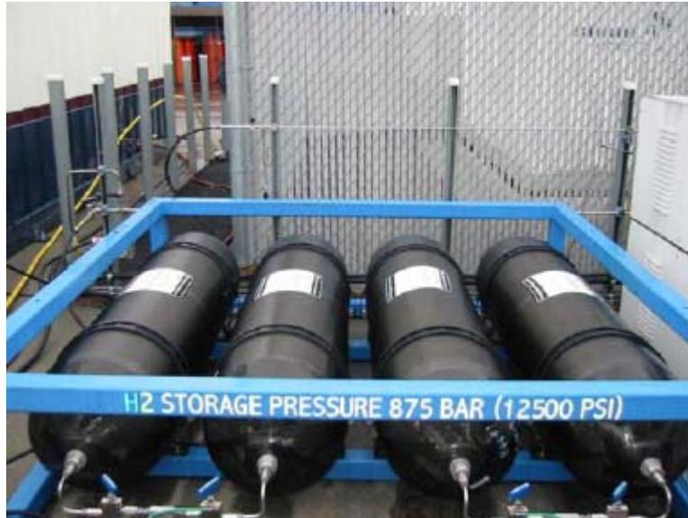
**Figure 6: Stationary storage – 875 bar carbon composite cylinders. Steel cylinders of equivalent capacity would be approximately 3 times the weight of the composite cylinders.**
