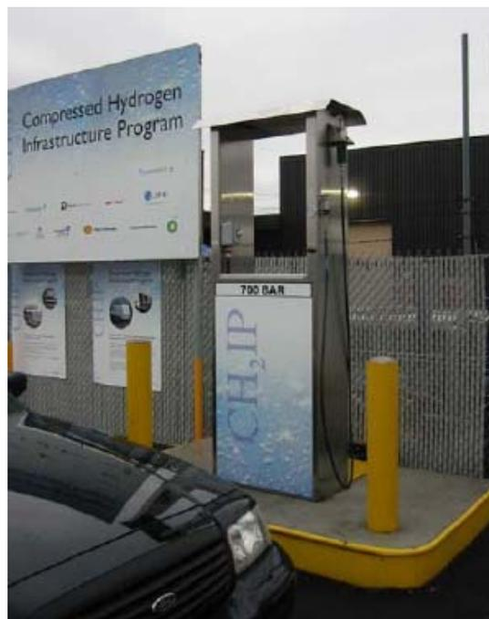
**Figure 7: Manual 700 bar dispenser. All the components including valves, nozzles, and hoses were rated to operate at 875 bar and were tested at Powertech prior to installation**
