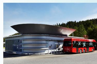
The Hynor Lillestrøm HRS opened in Lillestrøm in 2012. It also functions as a national test centre for demonstration of new HFC technology. The companies ZEG Power and Hystorsys are testing hydrogen production from reforming of locally produced biogas as well as metal hydride storage, in collaboration with the Institute for Energy Technology.
