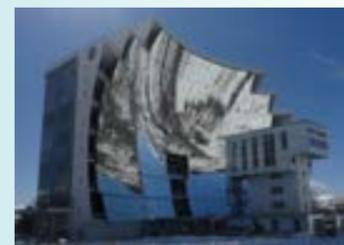
Figure 1: 1 MW solar furnace (MWSF), Odeillo, France, consisting of heliostat field, parabolic concentrator, and tower with experimental platform, which is used with the 100 kW solar pilot reactor to produce Zn.
